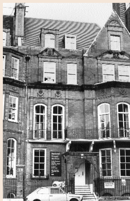
The NSA's former home in South Kensington
