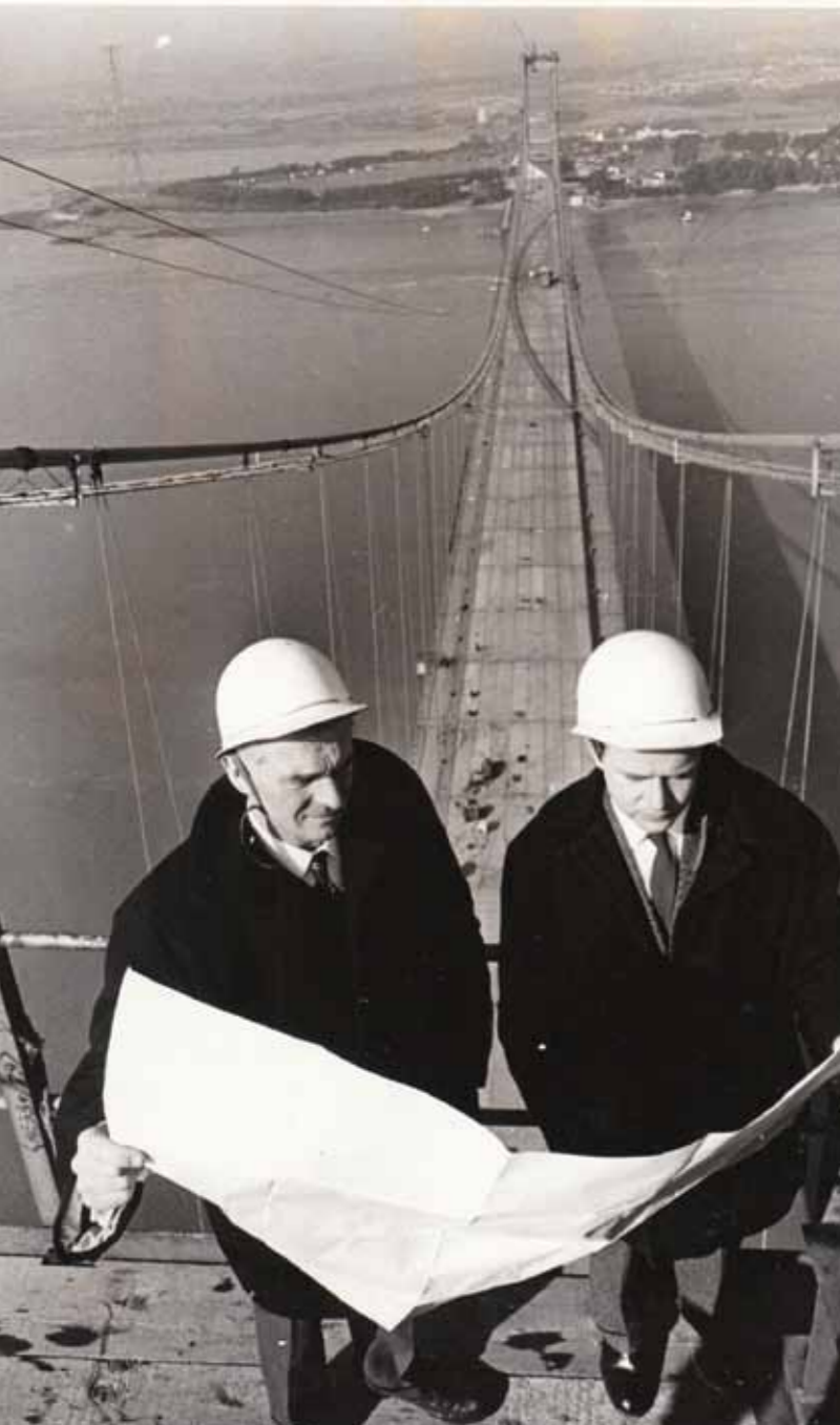
Michael Parsons (right) atop the Severn Bridge during construction, 1960s.
